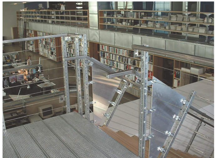
Unistrut Railing for Stairs and Walkways
