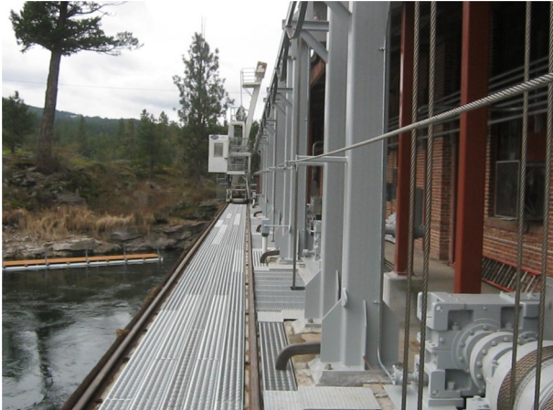
Horizontal fall protection lifeline at dam
