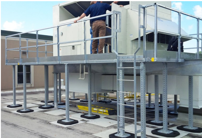
Rooftop walkway grating & platform to access mechanical unit
