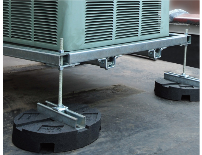
Rooftop Equipment Support
