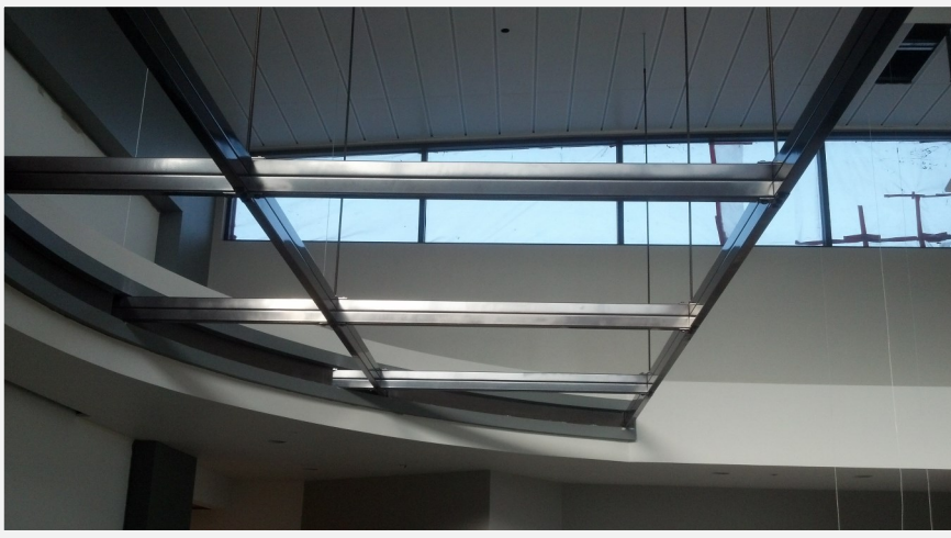
Powder coated ceiling grid in foyer
