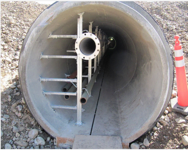
Unistrut in underground pipe/utility tunnel
