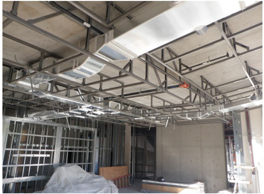
Architectural grids in University lecture hall before completion
