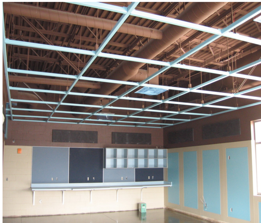
Ceiling grid in YMCA
