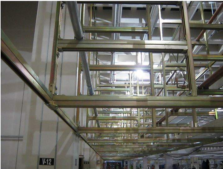
Close-up of installed Unistrut frames
