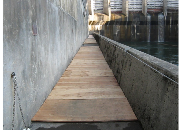
Horizontal fall protection lifeline at dam
