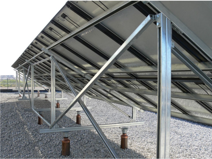
Solar Panel Framing
