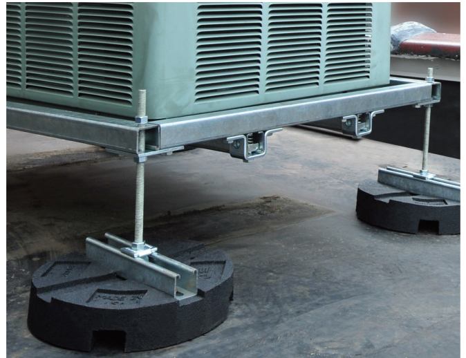
Rooftop Equipment Support
