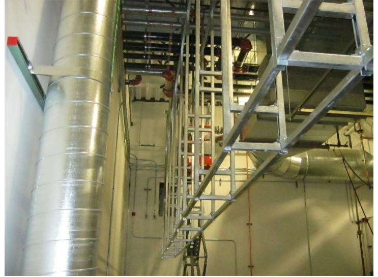
Assembled Unistrut frames for piping & conduit installed in manufacturing facility
