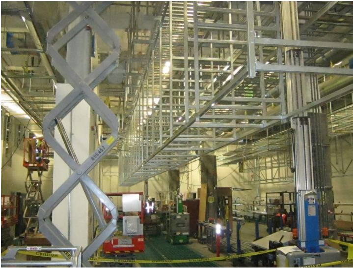
Assembled Unistrut frames for piping & conduit installed in manufacturing facility
