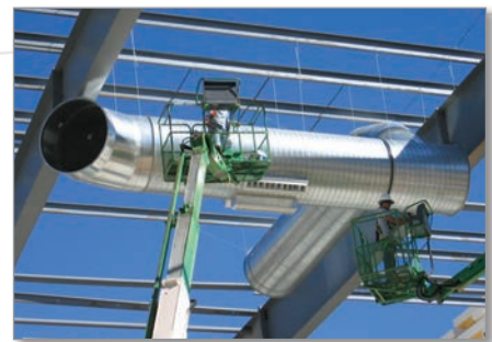
Gripple in the Construction industry
